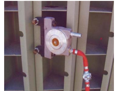
Turbine vibrator with a flange mount bracket on a staircase form.
