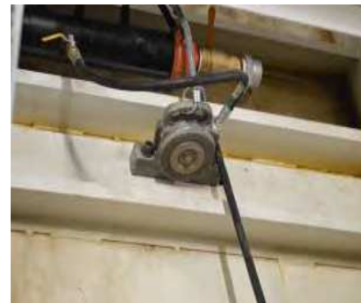
Model DTV-3 vibrator being used on a tunnel form.
