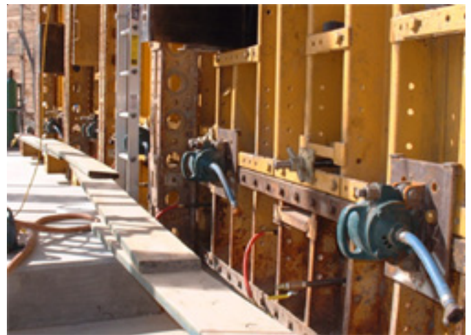
Roller vibrators on a wall for a water storage tank.
