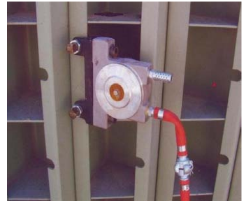
Model DTV7-3 vibrator with a TVMC clamp-on bracket on a staircase form.
